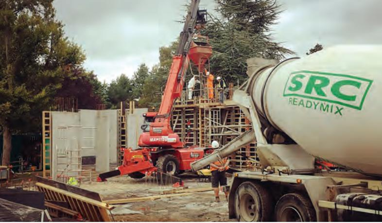
Concrete placement for rear wall to garden using 360° telehandler and concrete skip.
